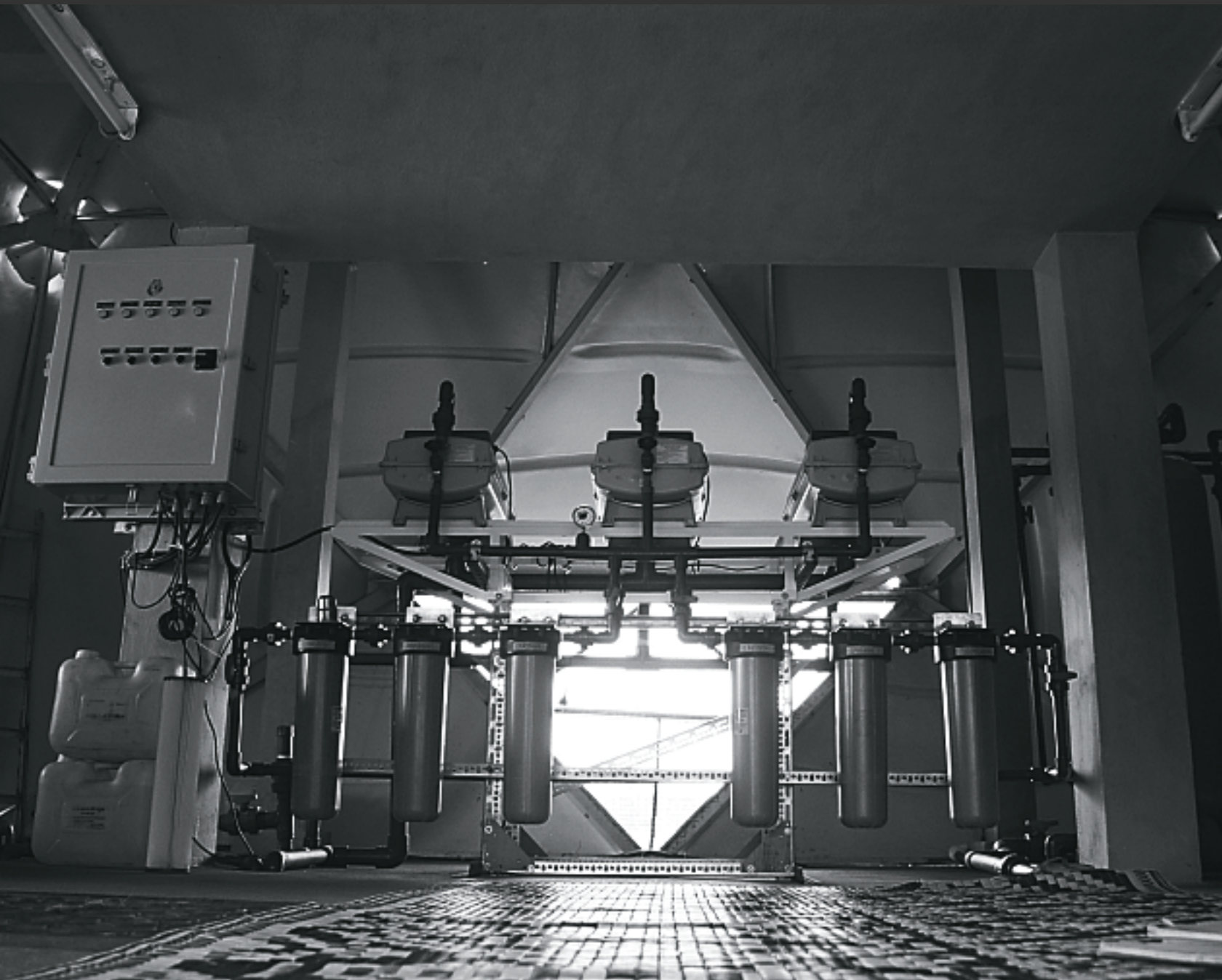
Interior of the Community Safe Water Plant at Bomminampadu that houses the UVWaterworks™ – the water disinfection system along with the multimedia, micron and carbon filters
